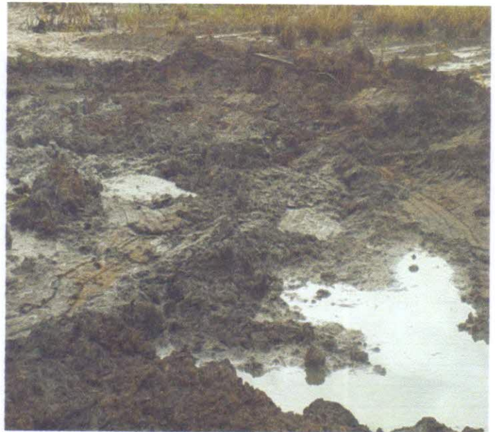
FIG.4 SHOWING SPILL POINT (AFTER BACK FILLED)
